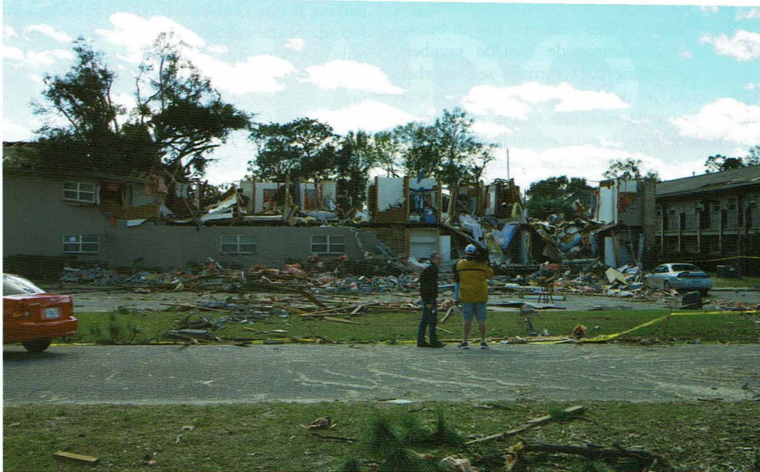
EF3 damage to an apartment building in Pensacola, Florida, in February.
