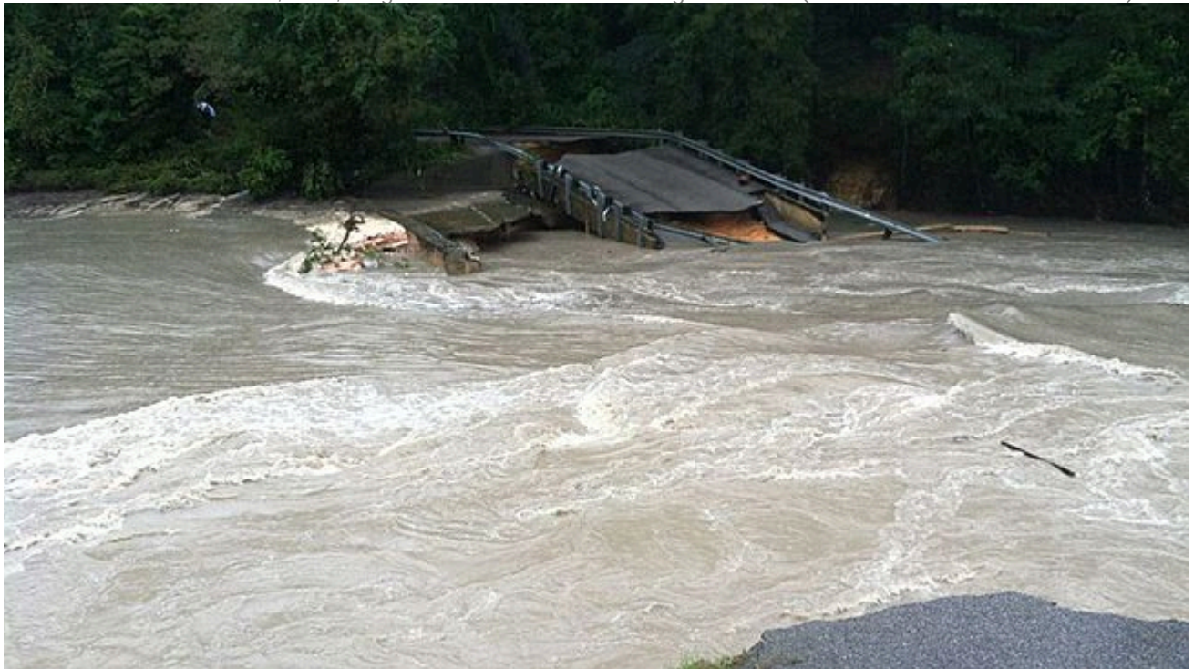
The Cary Lake Dam in the Columbia, S.C., area washed out on Sunday. (Facebook Photo/Gills Creek Watershed Association/Erich Miarka)
