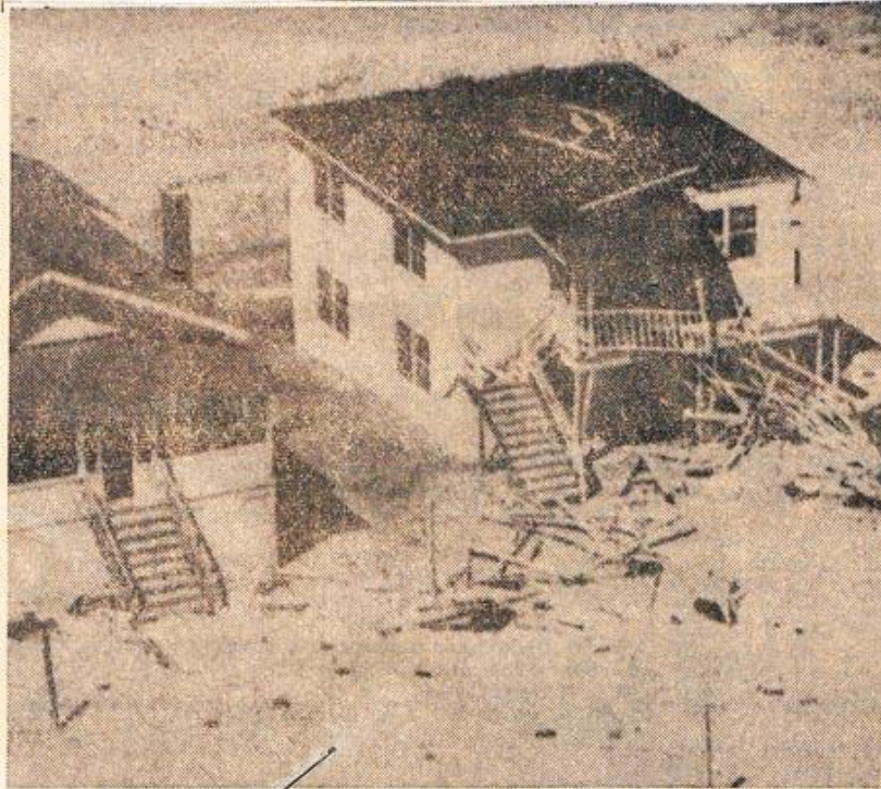
HURRICANE DAMAGE — This aerial photo shows one of many cottages damaged Saturday as hurricane Helene struck her heaviest blow in Carolina Beach, N. C. Property damage run in the millions on the North Carolina coast. (AP Wirephoto)
