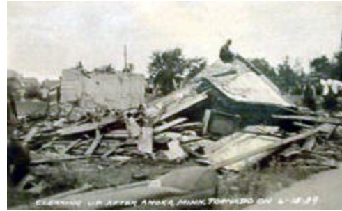
Cleaning Up After the Tornado, '39
