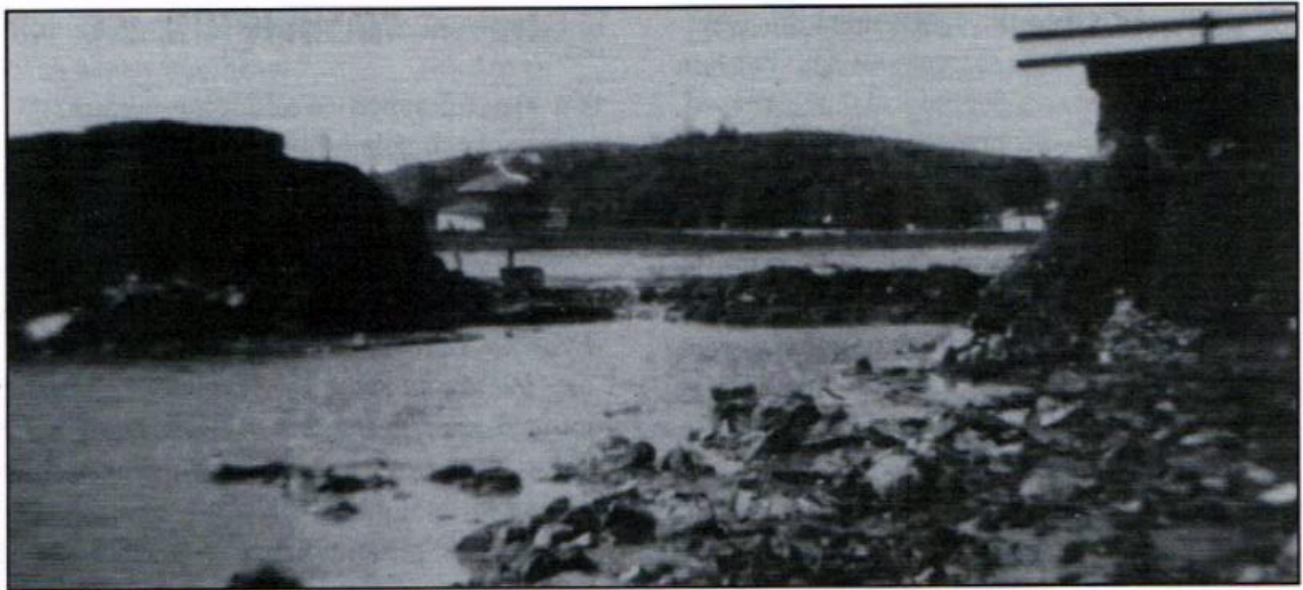
Water swept through Staunton, Va., after the failure of this dam on the edge of town. The torrent wrecked part of the business district.
