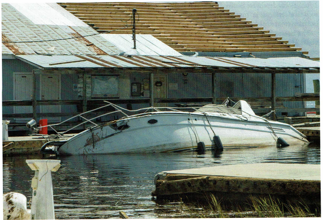
Damage at a pier in St. Mary's, Georgia, from Hurricane Irma, on September 23.
