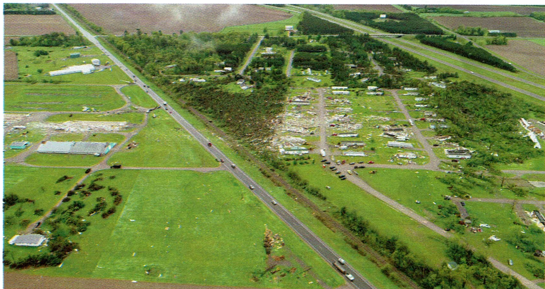
Severe tornado damage to a mobile home park in Chetek, Wisconsin, on May 16.
